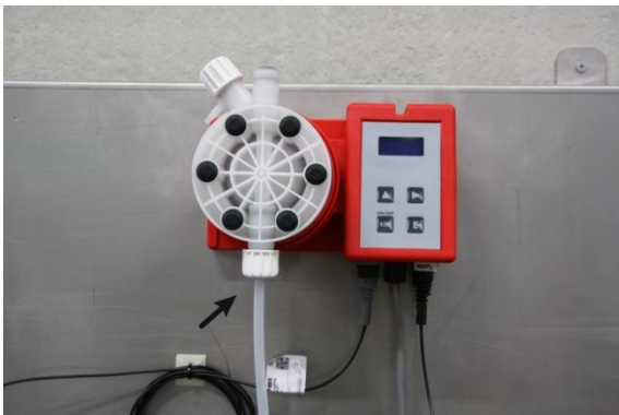
Figure 3: Connecting the suction hose
