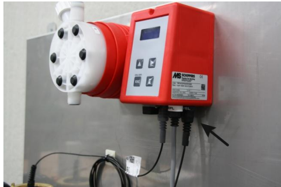
Figure 2: Connecting the dry-run protection
