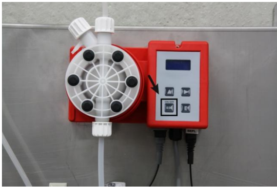
Figure 5: Switching the pump on
