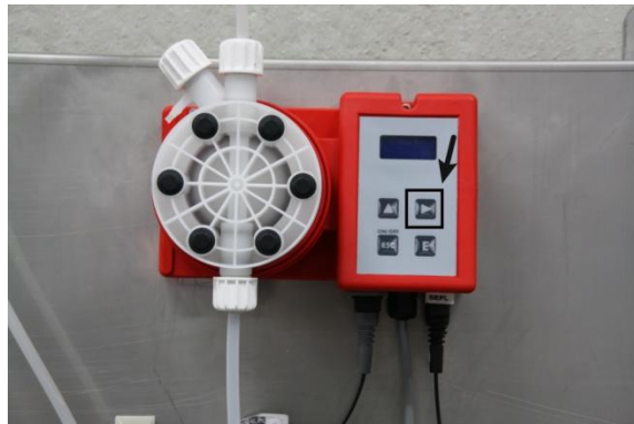
Figure 8: Filling the pressure hose
