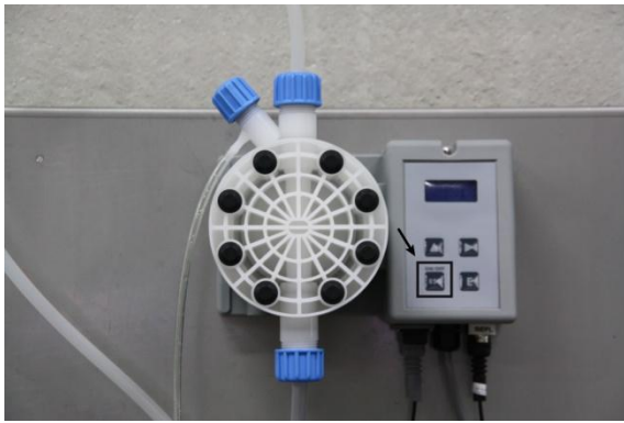
Figure 5: Switching the pump on
