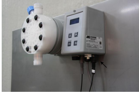
Figure 2: Connecting the dry-run protection and watermeter
