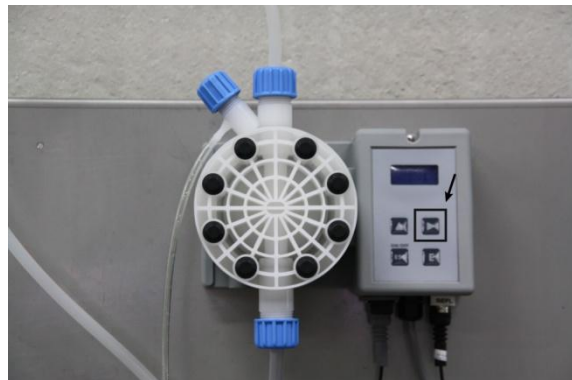
Figure 16: Filling the pressure hose
