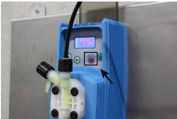
Figure 9: Switching the pump on
