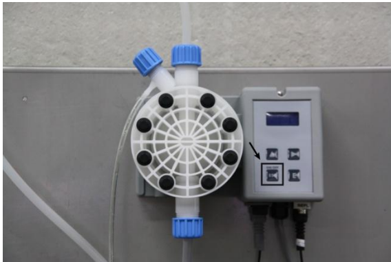
Figure 13: Switching the pump on
