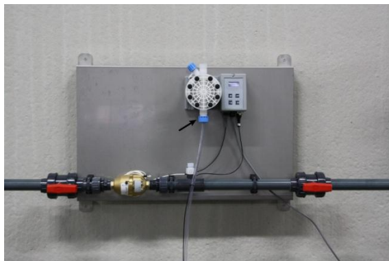
Figure 7: Connecting the suction hose
