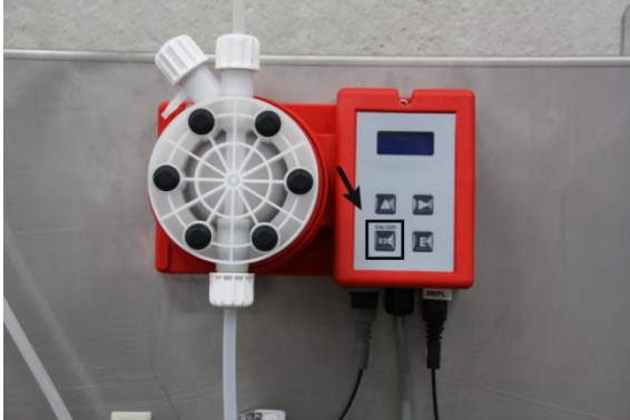
Figure 12: Switching the pump on
