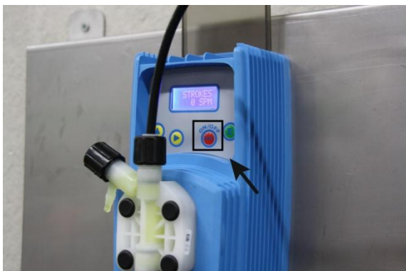
Figure 8: Switching the pump on
