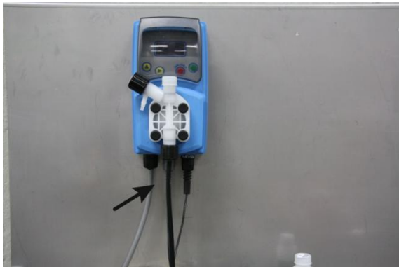
Figure 3: Connecting the suction hose
