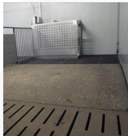
Sideways in the pen Allow sufficient space for easy entrance and exit, even when animals are heavier
