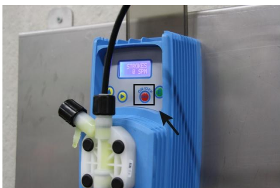
Figure 5: Switching the pump on
