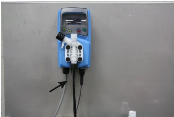
Figure 3: Connecting the suction
