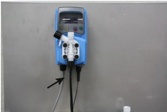
Figure 3: Connecting the suction
