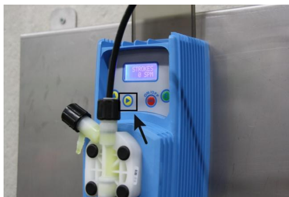
Figure 8: Filling the pressure hose
