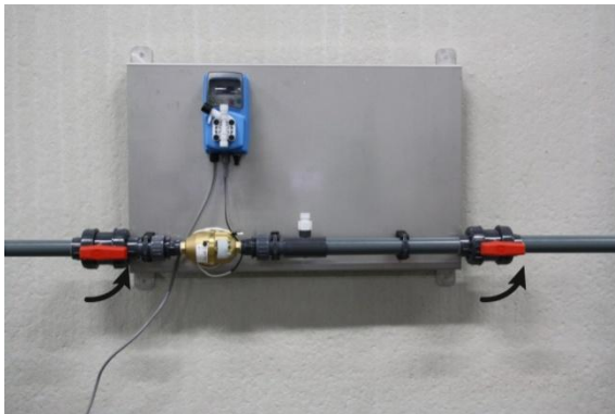
Figure 1: Open the ball valves
