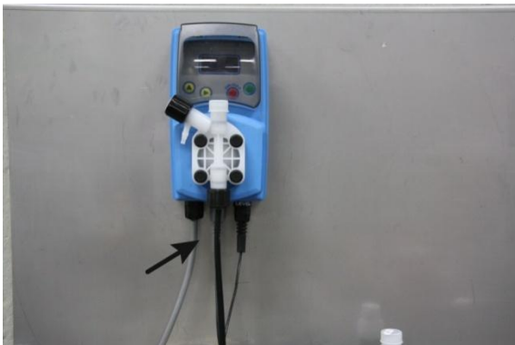
Figure 3: Connecting the suction hose
