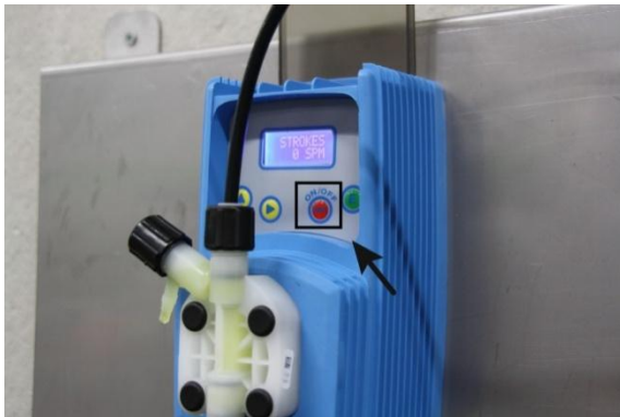
Figure 5: Switching the pump on
