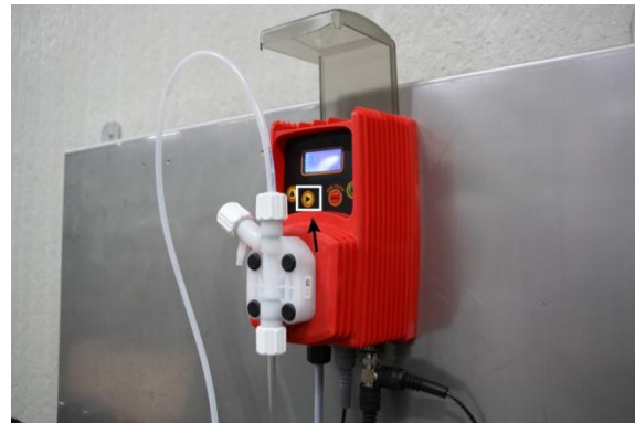
Figure 8: Filling the pressure hose
