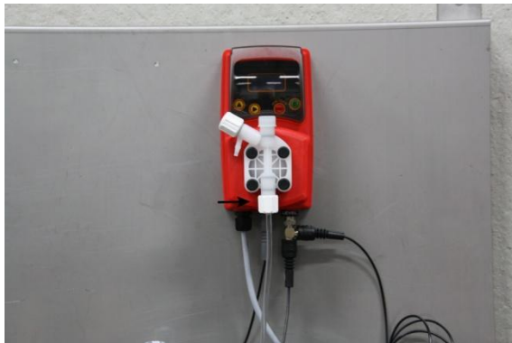
Figure 3: Connecting the suction hose
