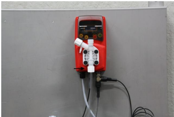
Figure 7: Connecting the suction hose
