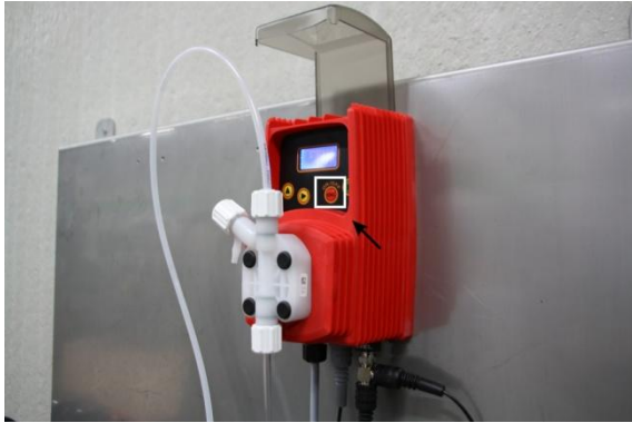
Figure 13: Switching the pump on
