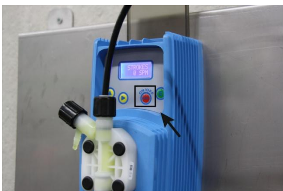
Figure 9: Switching the pump on
