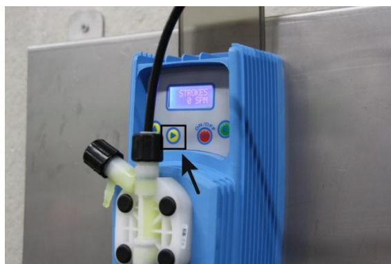
Figure 12: Filling the pressure hose
