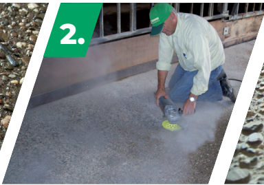
Sand the floor if needed
