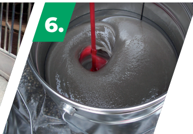
Mix components A and B
